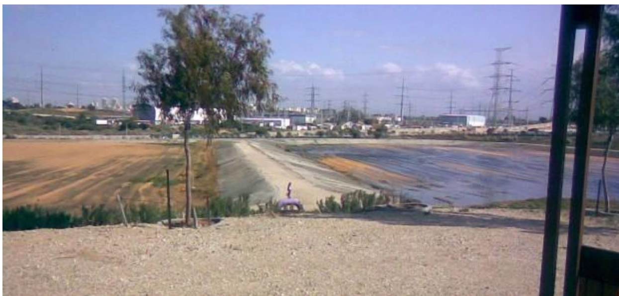
Fig. 4.4: Spreading basins drying and flooding at recharge site Soreq 2 of the Shafdan plant.
